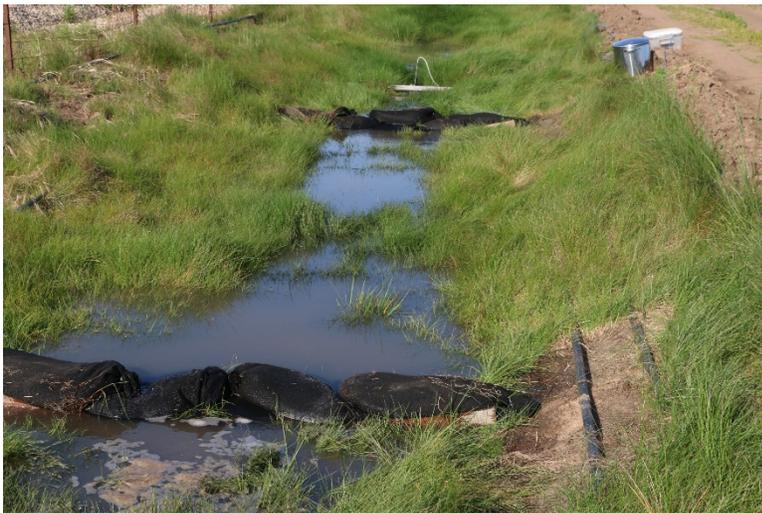
**Figure 2.** Carbon filters located at the lower end of the vegetated ditch.
